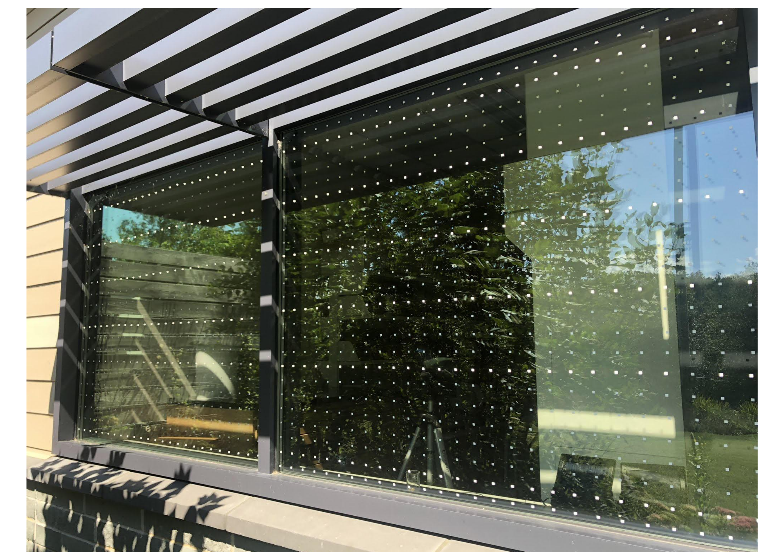
Figure 4: Feather Friendly ® stickers applied by volunteers to the windows of Rice Creek Field Station
