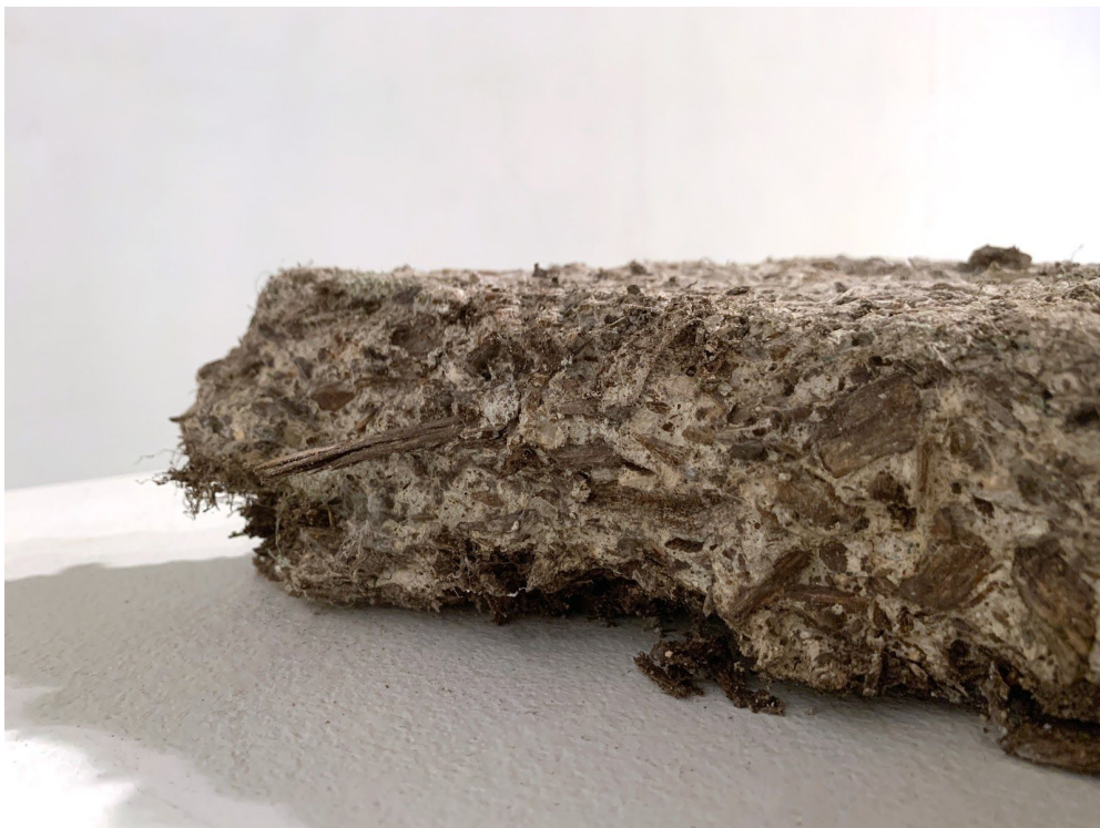
(Figure 4, edited white balance) Two weeks post concrete, broken chunk of slab from deinstallation
