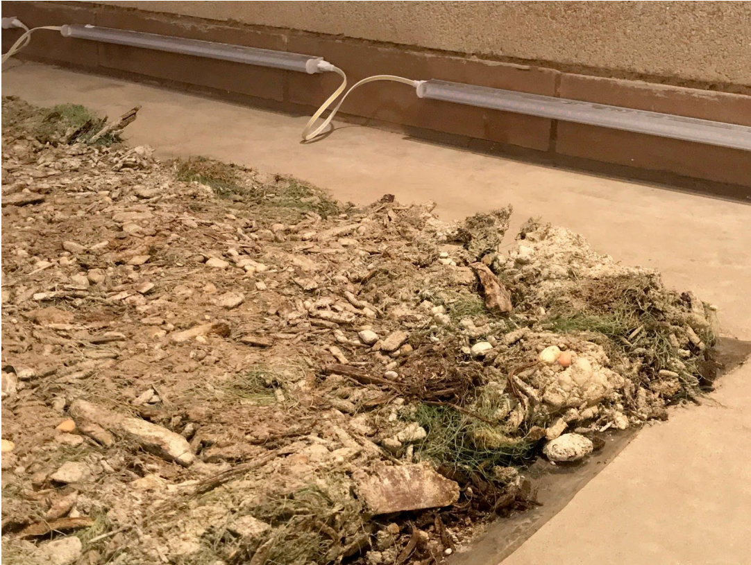
(Figure 1, taken in the bad Barn lighting.) Two days post concrete, left corner
