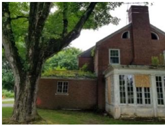
Figure 10: Fairfield Hills Hospital in decay, Newtown Ct. Closed in 1995, now hosting flora and fauna.
