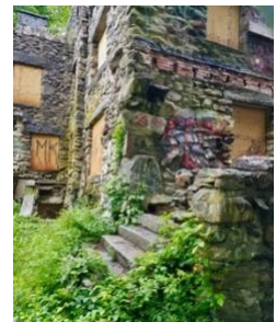
Figure 9: Hearthstone Castle in Danbury, Connecticut. Interior roofs collapsed; the forest is taking over.
